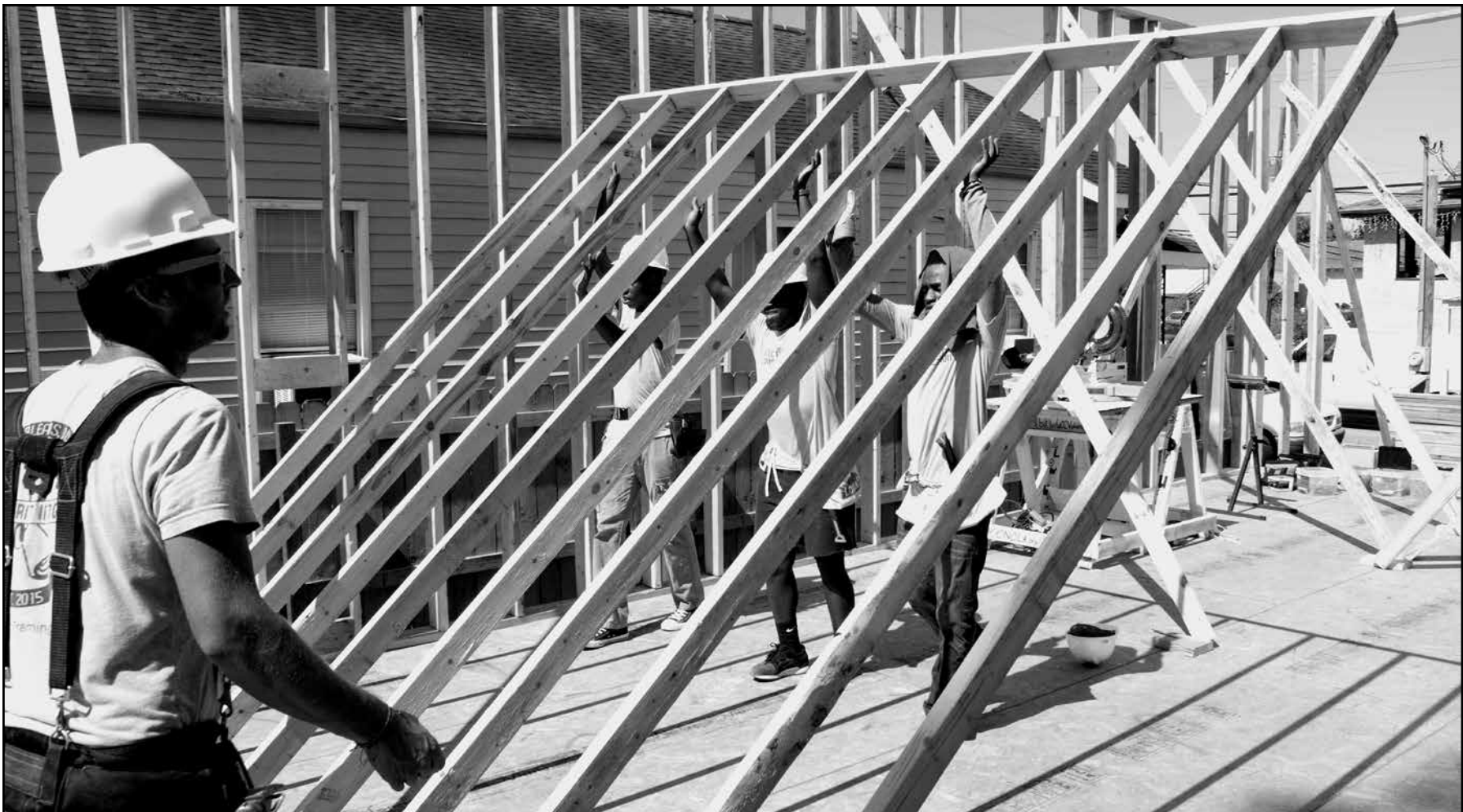
Students lift 12 foot interior wall that is ready to install.
